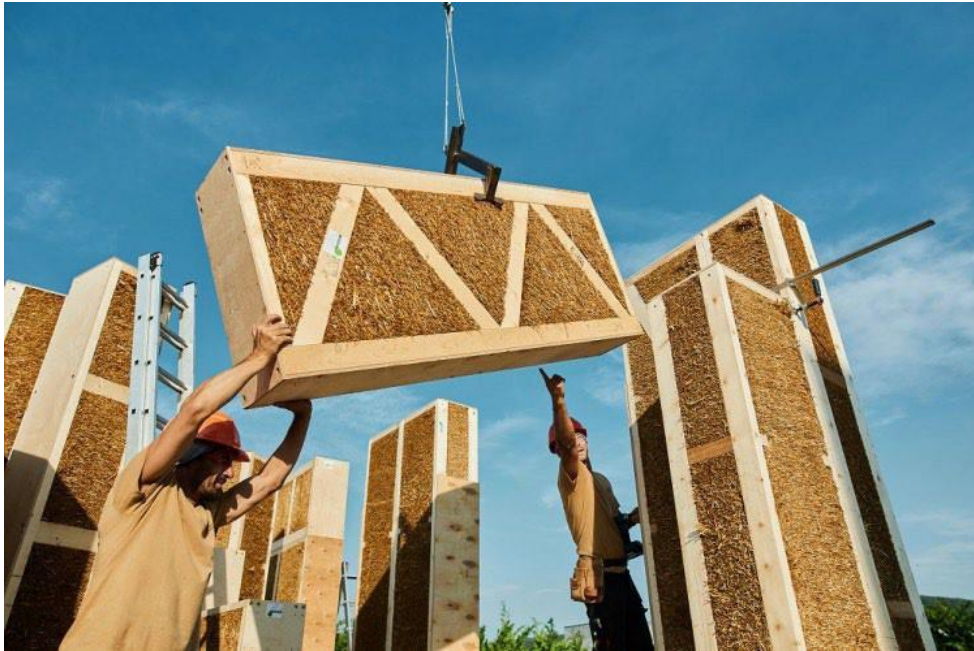
EcoCocon, compressed straw cassette assembly, 2022
