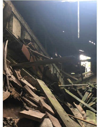
Fig 2. North Wing Interior
