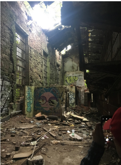
Fig 5. East Wing Interior
