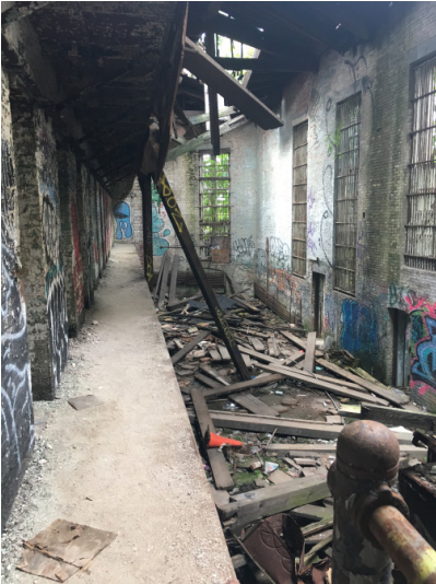
Fig 2. West Wing Interior
