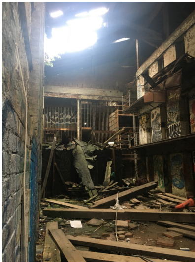
Fig 6. East Wing Interior
