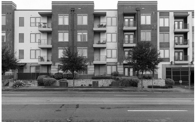
The now ubiquitous “stick-frame-over-podium” building type.
